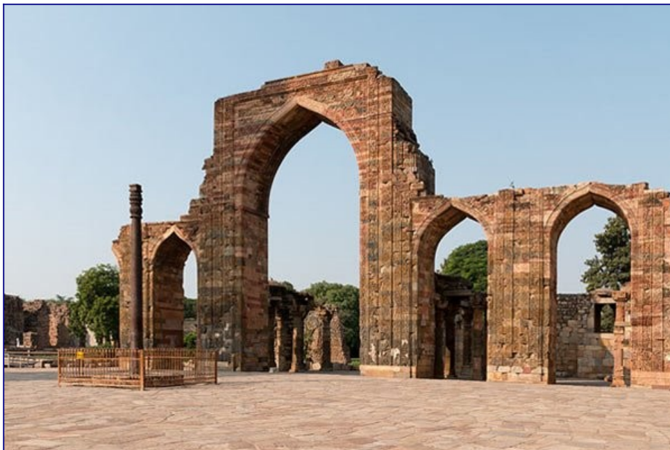
The Incredible Rust-Resistant Iron Pillar of Delhi
